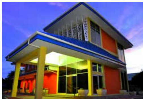
■ The new Family Development Research Centre.
