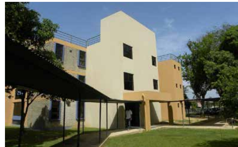
■ The front entrance of the refurbished South Block at Canada Hall.
