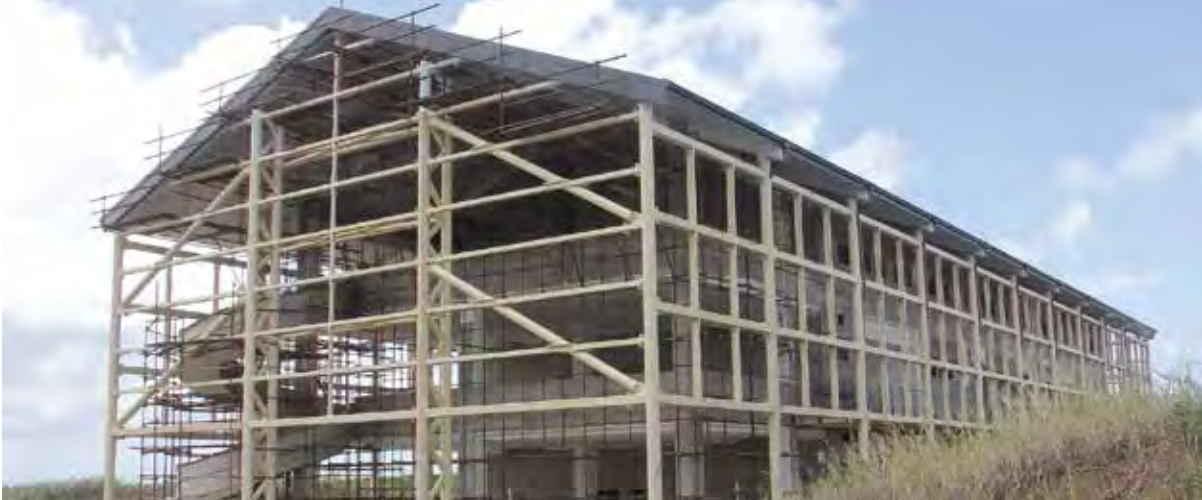
Construction at the new South Campus at Penal/Debe
