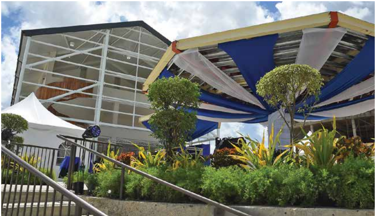
Part of the completed construction at The UWI St. Augustine South Campus, Penal/Debe.
