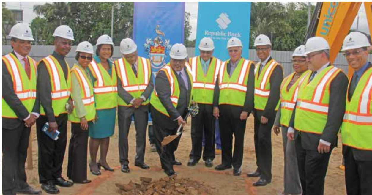
Executive Director, Republic Bank Ltd., Mr Derwin Howell, turns the sod for the UWI-Republic Bank Plaza as executives from both organisations look on.
