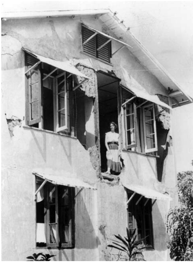
Katz house on Santa Margarita Circular Road, St. Augustine damaged in the 1954 earthquake off the north-west coast of Trinidad. (Photographer: Dr. G.R. Robson)
