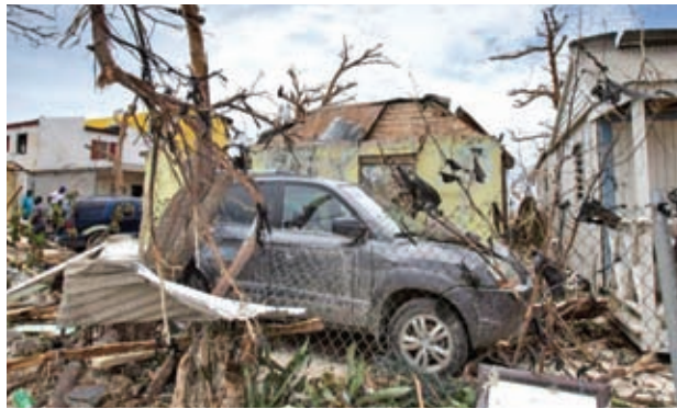
Storm damage from Hurricane Irma is seen in St Martin, Sept. 7, 2017 PHOTO: THE DUTCH DEFENSE MINISTRY
